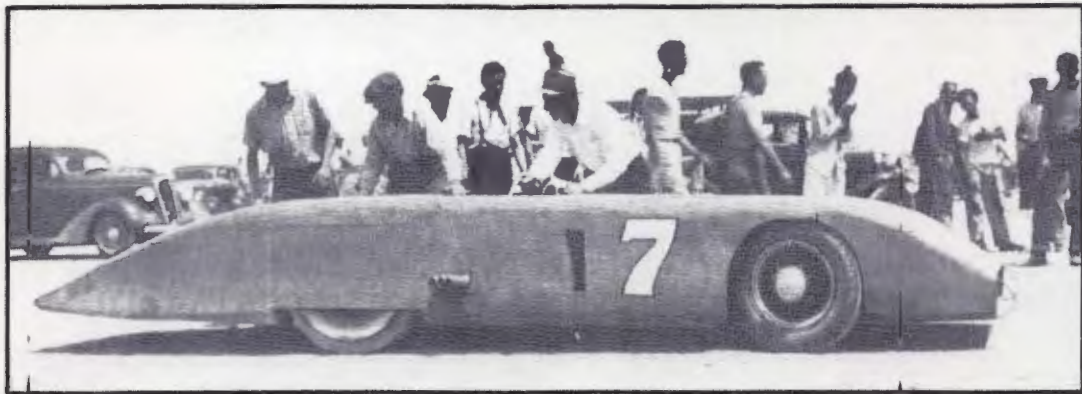
This is the first full-envelope record car made in America and perhaps the first V-8 lakes entry to run methanol—the Spalding Brothers famous streamliner. Engine was bored-out 21-stud with Harman cam, milled heads, and the Spaldings' own manifold and ignition. The car officially ran 128.75 mph in 1939 and
